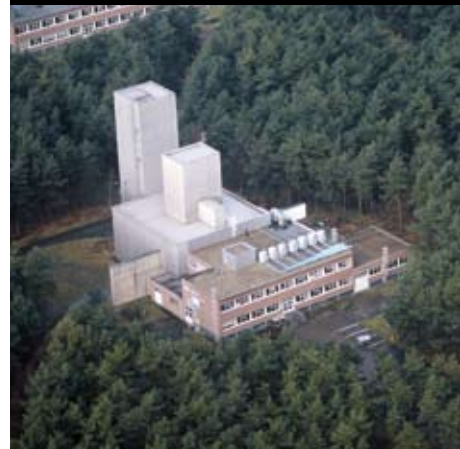
Aerial view of the Van de Graaff building, showing the two towers housing the 3.7 MV and the 7 MV machines.
