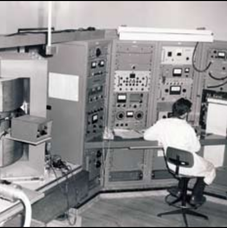
A Nuclide Tandem isotope mass spectrometer (Nuclide Corporation, State College, PA, USA).
