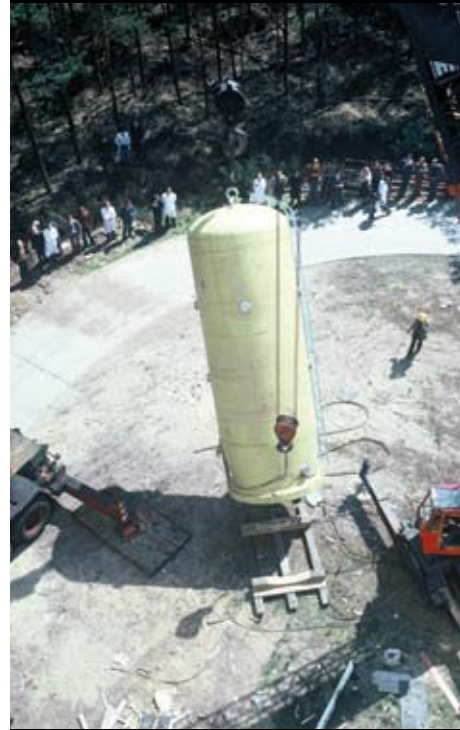
Installation of the 16-ton, 7 MV Van de Graaff accelerator (29 April 1976).
